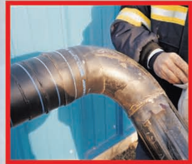
Ideally suited for uninterrupted application to elbows and straight lengths of pipes.
