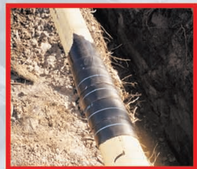
Pipes protected with tape sealant can be used above or below grade.
